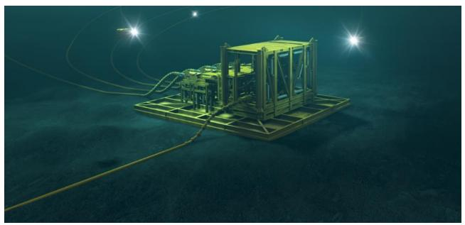
Figure 8-25: Subsea Transformer Station with incoming cable from shore (front) and outgoing cables to FPSOs (back). Here shown with 4 output cables, two to each FPSO
