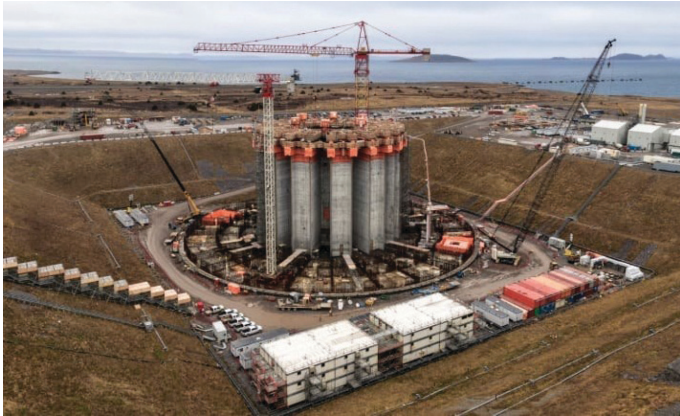
Concrete Gravity Structure under construction at Argentina. Photo courtesy of Husky Energy.
