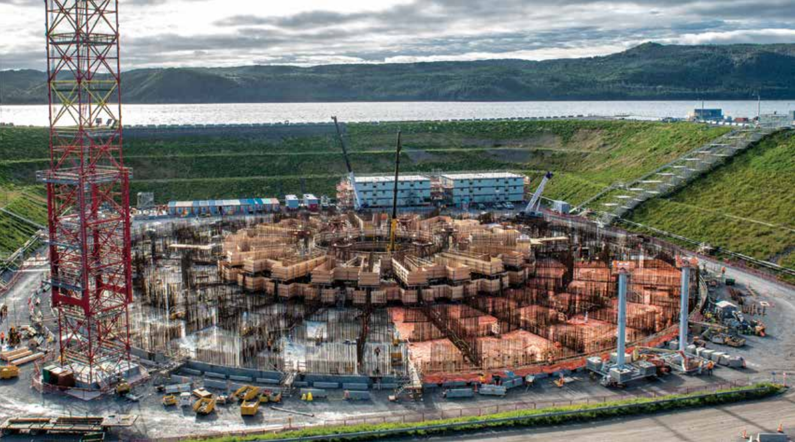
Construction of the West White Rose concrete gravity structure continues at Husky Energy's Argentia graving dock site.
